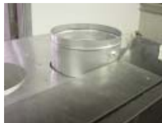
Fig. 4 -Insert Starter Plenum all the Way into opening
