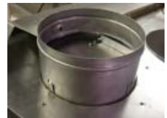
Fig. 5 - Fasten 3 tabs to top of fireplace
