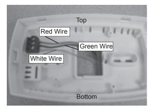
Figure 20.1 - Back Side of Wall Control with Cover Off
